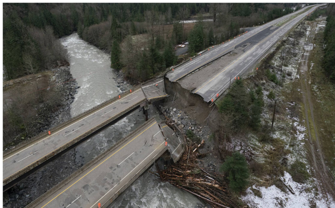
Damage to the Coquihalla Highway from the 2021 BC flooding
